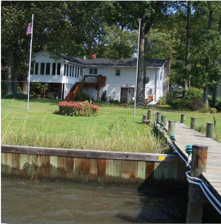
This study site represents a typical Chesapeake Bay residence where the drainfield is located in the back yard adjacent to the Bay.
